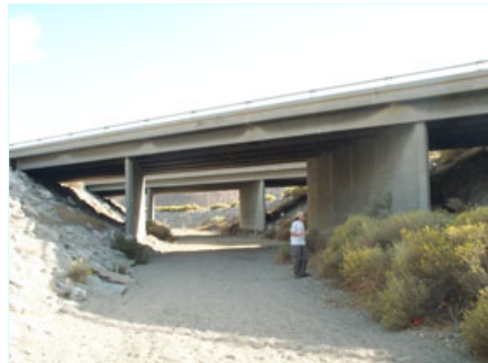
Figure 35. The north side of SR 58 at Sand Creek.
