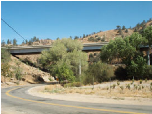
Figure 34. SR-58 bridge over Tehachapi Creek. The paved road connects the east and west portions of Keene.
