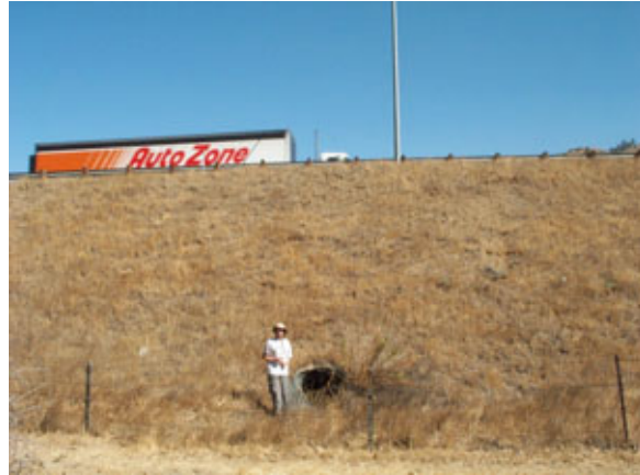
Figure 32: Fill slope along SR-58 that should be replaced with a bridge.
