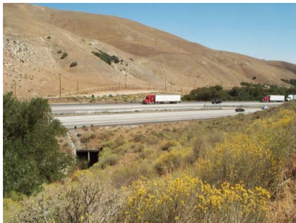
Figure 31. Culvert on Interstate-5 for Gorman Creek with Hungry Valley State Park in the foreground. Note steep degraded slopes on far side of I-5.
